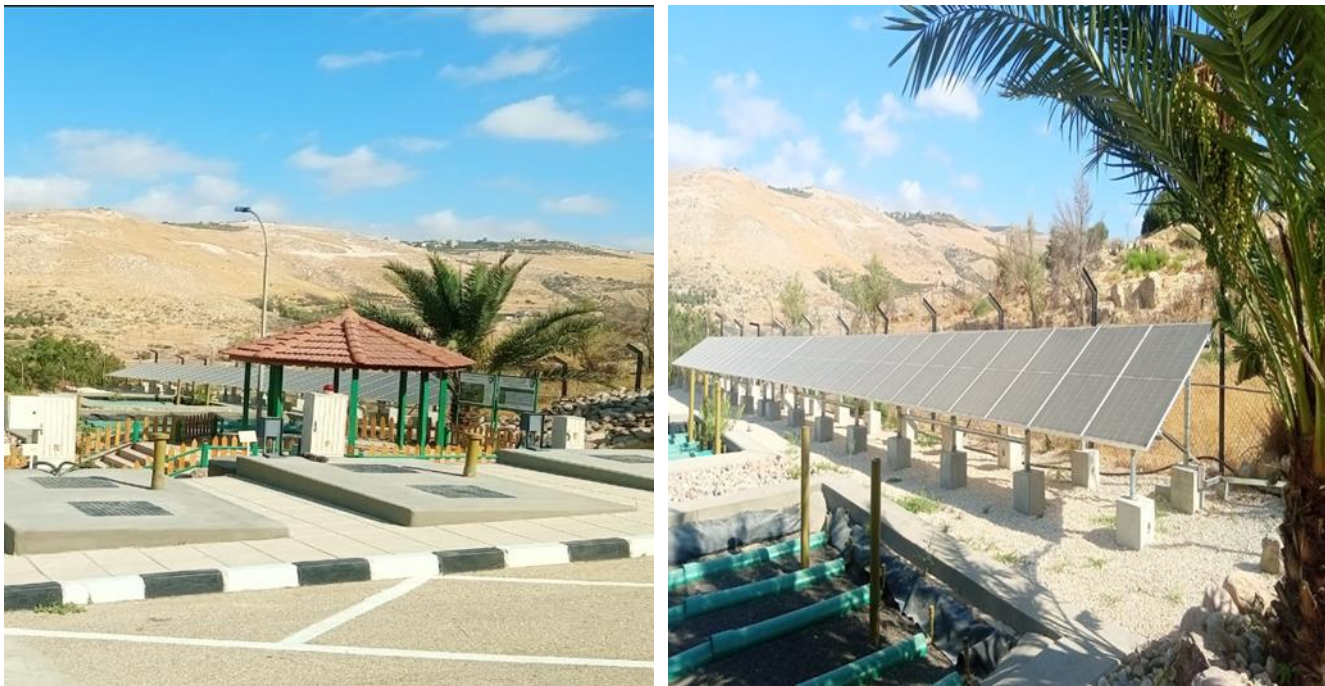
Solar panels at BAU
